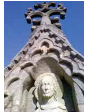
Restored stonework on the West Front
