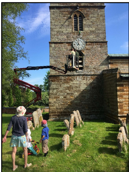
Removal of the clock face for repair
